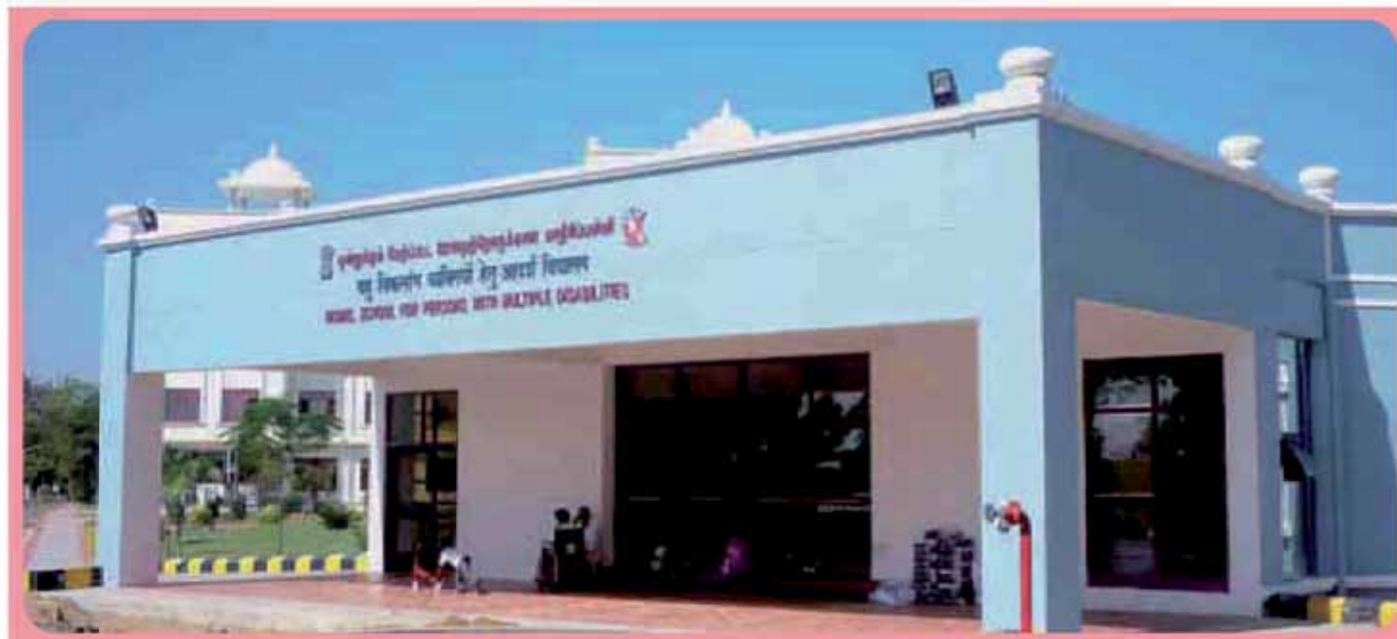
View of the Model School building
