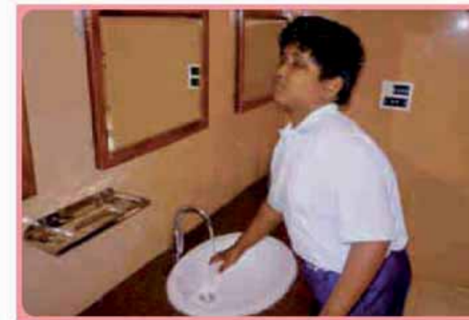
Sensor based washbasin for easy handling
