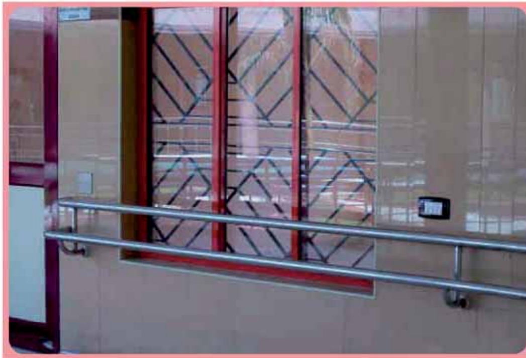
Doors and windows with bright colored paints
