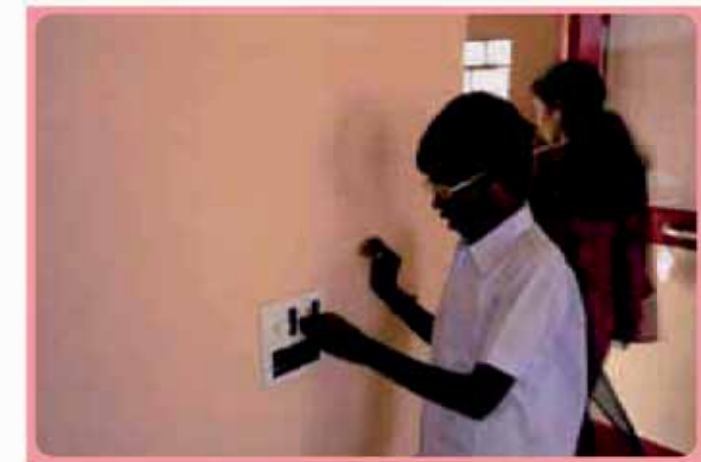
Switches installed at suitable height with Braille Inscription
